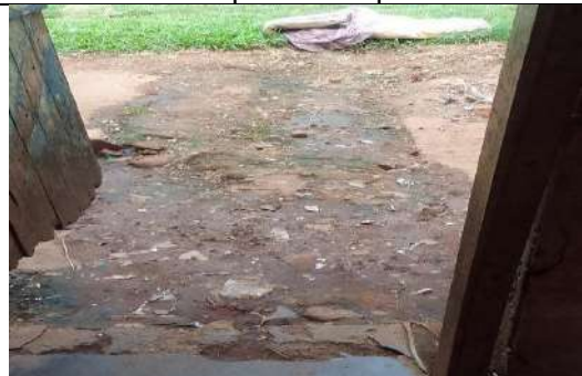
Iganga Hospital: Entrance to the inpatient bathrooms.
