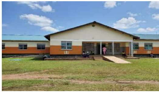
R- Newly constructed maternity block at Koch Li HCIII
