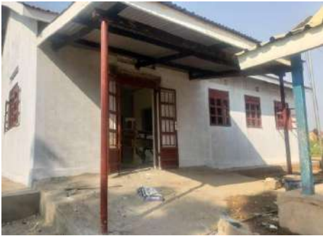
OPD block construction at Buyende HCIII.
