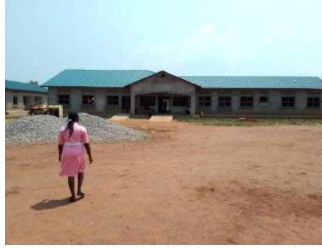
Ongoing expansion works at Bukungu HCII
