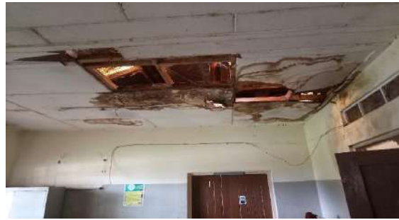
Status of some structures in Grade A-
