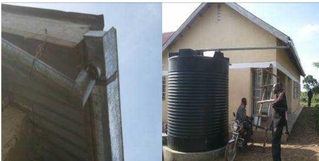
*A non functional system clogged with leaves in Muduma HCIII despite the tank being in good condition.*
