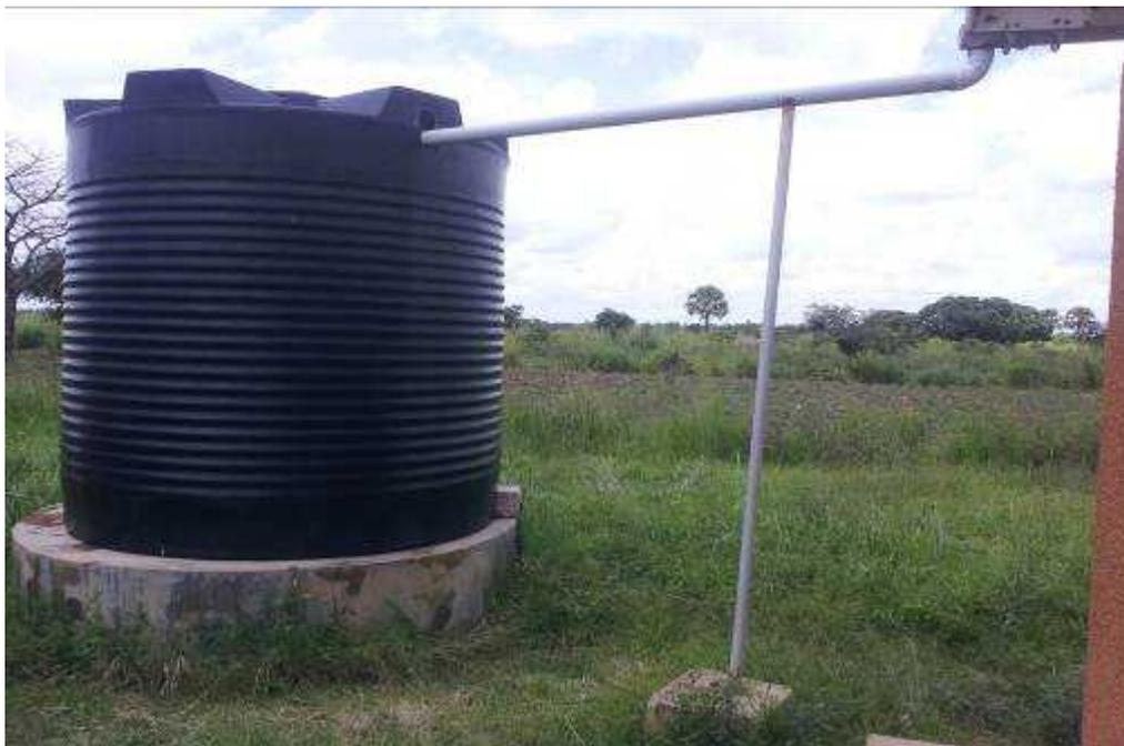
*Well constructed and functional water harvesting system at Aromo HCIII*
