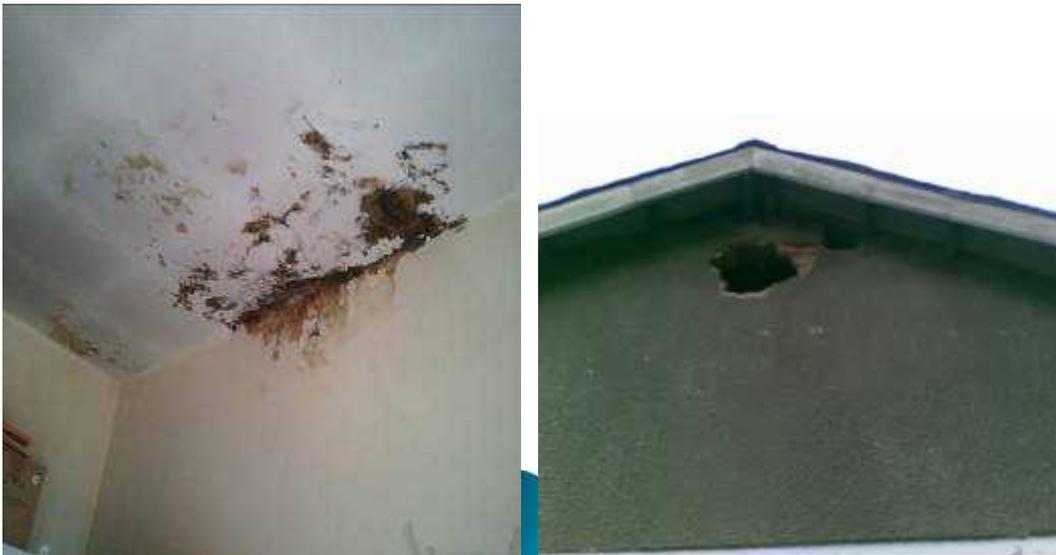
*Bat urine and faecal matter causing extensive damage to cement ceiling at Kyai HCIII and roof of Buyanja HCII*
